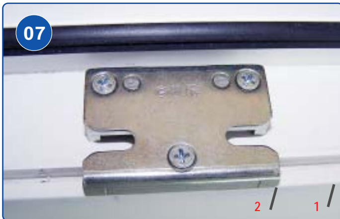
INSTALL BOTTOM TILT KEEPER AT BOTTOM OF FRAME AND FASTEN WITH TYPE "D1" SCREWS
