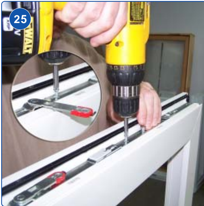
FASTEN STAY ARM FACE PLATE INTO POSITION FASTENING SCREW BEHIND CLIP OF STAY ARM FACE PLATE
