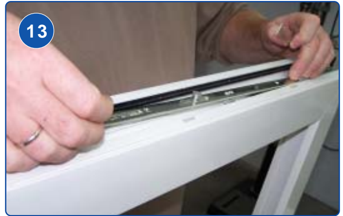
13 PLACE GEAR BETWEEN CORNER TRANSMISSIONS • Use handle to center in turn position
