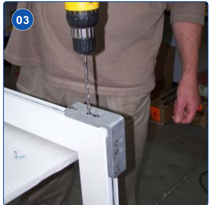
DRILLING FOR HINGE BEARING AT BOTTOM OF SASH
