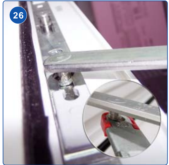
ATTACH END OF STAY ARM (LEFT/RIGHT) TO STAY ARM FACE PLATE AND CLIP STAY ARM LINK ONTO MOUNT OF STAY ARM FACE PLATE
