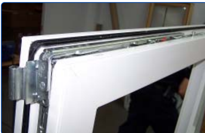
LIFT STAY ARM OVER SLIDE CAMS OF FACE PLATE INTO CLOSED POSITION
