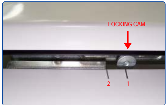
LOCKING CAM AND KEEPER ARE IN GOOD POSITIONS
