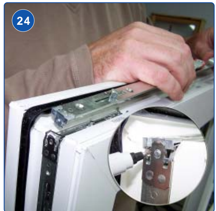
24 CLIP STAY ARM CONNECTING PLATE ONTO MID-LOCK END OR ALIGN STAY ARM CONNECTING PLATE FLUSH TO CORNER
