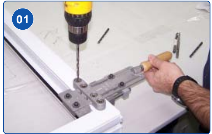
DRILLING FOR BOTTOM HINGE
