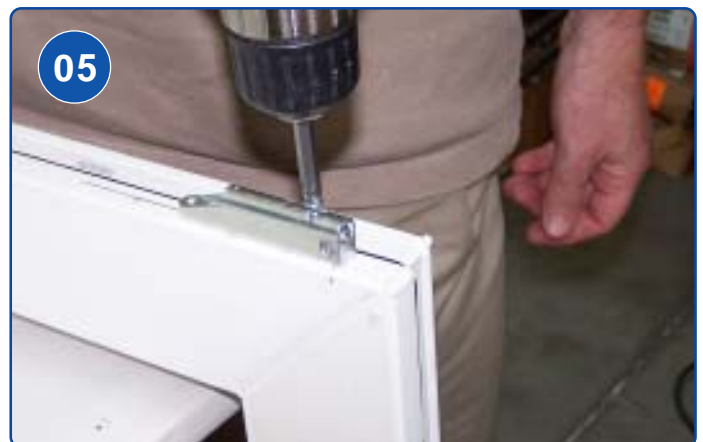
FASTEN WITH TWO 38 mm TYPE "D1" SCREWS E-12562-XX-0-1
