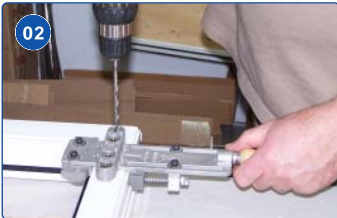
DRILLING FOR STAY ARM BEARING
