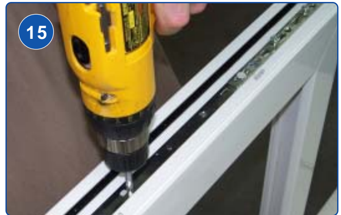
15 FASTEN GEAR IN PLACE WITH TYPE "D1" 25-30 mm SCREWS E-12562-XX-0-1
