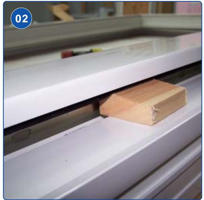
PUT SPACER BETWEEN SASH AND FRAME ON HANDLE SIDE FOR EASY ACCESS TO LOCKING CAMS
